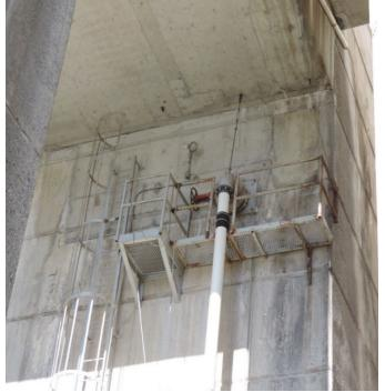
Figure 3-7. Closer View of the Existing Drain Valve for Diffuser 16.
