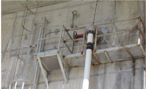
The diffuser drain pipe is located near EL 229 feet. The lamprey trap is located at EL 185 feet. This provides around 83 feet of head for the system to overcome friction losses due to valves and fittings. The drain pipe will be replaced with schedule 80 PVC piping. The existing air valve will be replaced with a combination air release and vacuum valve and moved further up the drainage pipe. The existing pipe supports will be re-used for the new piping.
